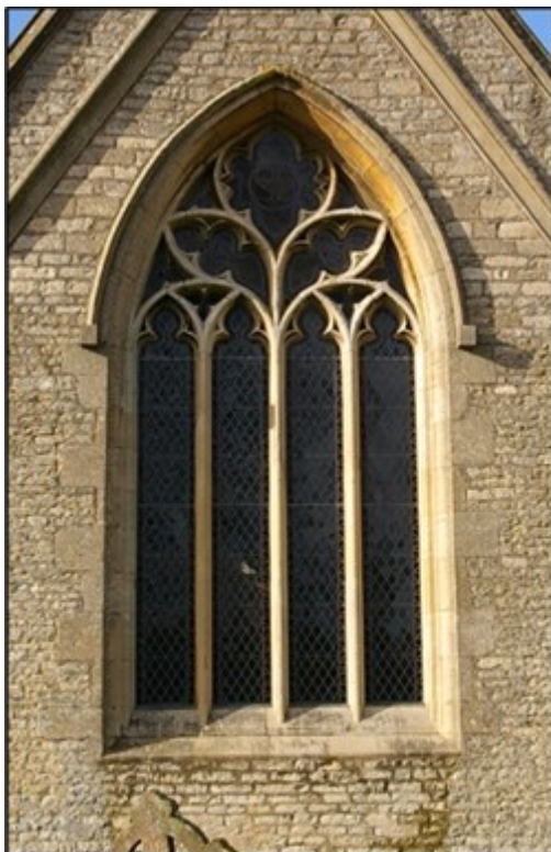
Swinstead east window Cusped curvilinear tracery. C14. Restored
