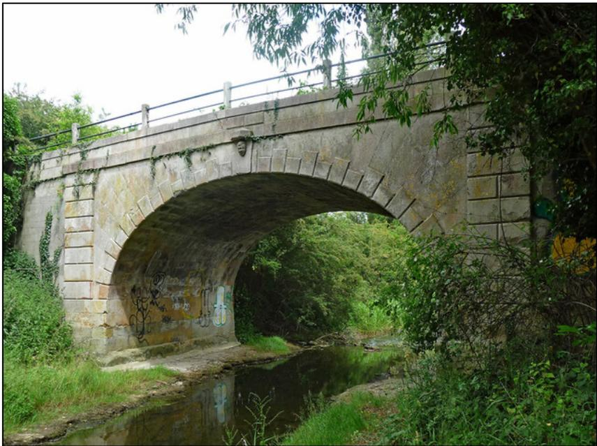
The bridge is late 18<sup>th</sup> century but appears to be in superb condition. It is a single elliptical arch. The stone blocks have smooth faces and sharp square edges. Either side of the arch are pilasters which are flat representations of classical columns. All masonry blocks on the pilasters and the arch on the east and
